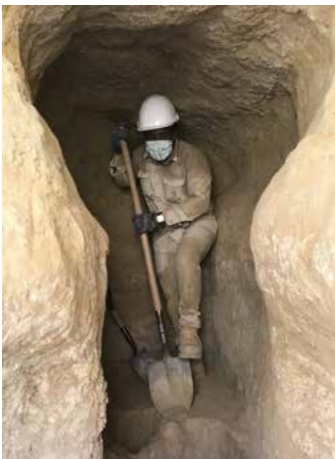
Hili Misbah. Excavation of a rock-cut tunnel in progress
