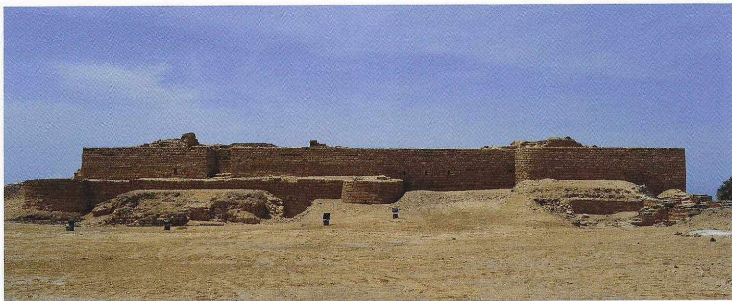
Fig. 1 – The northern side of Husn Al-Baleed after the consolidation work (Photo A. Pavan for the Office of the Adviser to His Majesty the Sultan for Cultural Affairs).
