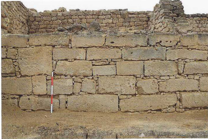
Fig. 4 – Wall 20/M90. Built with very large masonry blocks, it belongs to the first construction phase (Photo A. Pavan for the Office of the Adviser to His Majesty the Sultan for Cultural Affairs).
