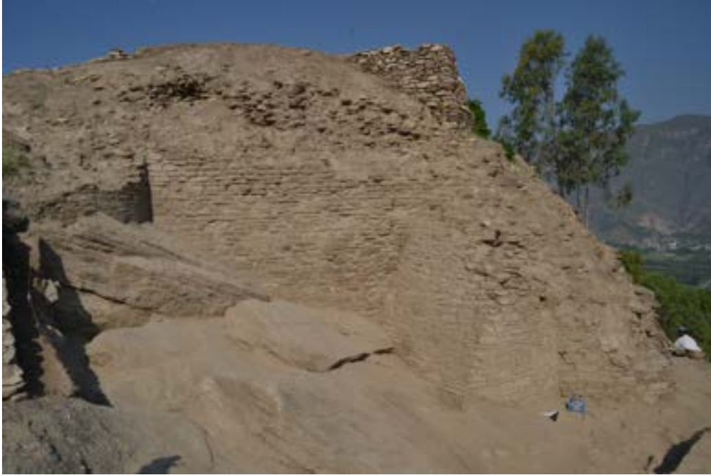
Fig. 7 – Counterfort 2 of the NE tower
