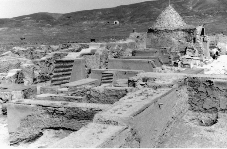
Fig. 5 - 1966. Protection and consolidation work in the south-western side of the Palace. (Dep. CS Neg. R 4417/6; © IsIAO).
