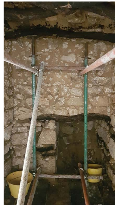
Fig. 10 - Consolidation works at the second storey of the citadel, June 2019 (Photo by A. Gratteri).
