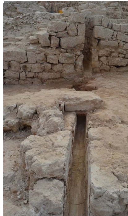
Fig. 40 - Draining channel crossing the western curtain wall.
