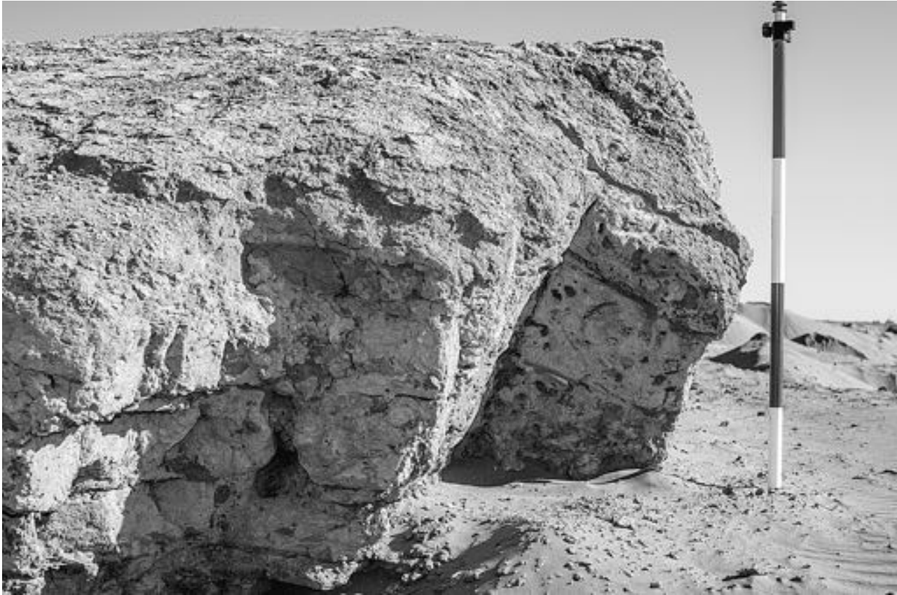
Fig. 14. Detail of the main vault between the plinths from the south (western plinth).
