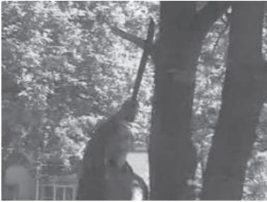
Cut off branch 97
