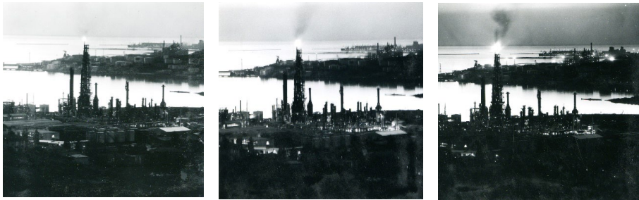
Figs. 10-12 – Alfonso Mottola, Night view with Ironwork plant , 1970?.
