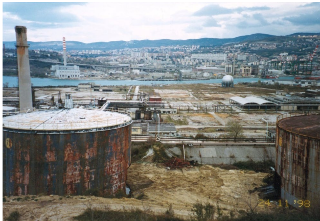
Fig. 8 – The Aquila industrial site at the end of the 1990s
