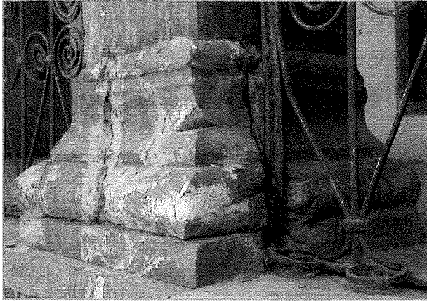
Fig. 2. Base of the loggia pillar
