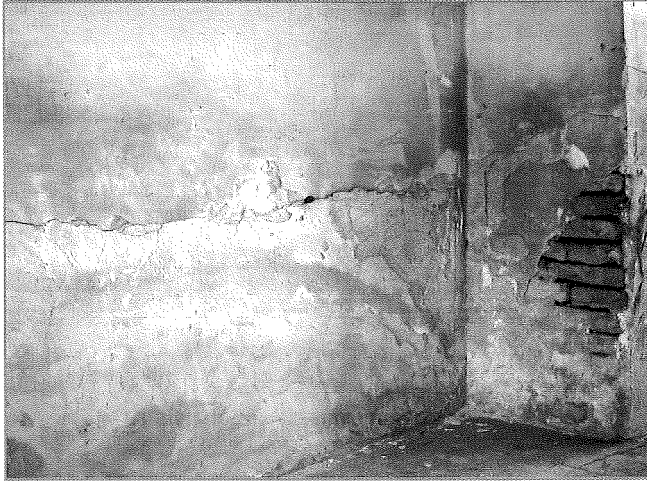
Fig. 3. Damage caused by water seepage on the SW wall, adjacent to B1-1/3 building
