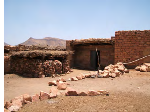
b) Traditional house in Liban ( ħədmə ). (Photo by G. Lusini).
