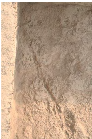
Fig. 12 - Trench no 5, an alignment of a possibly another wall SU41 perpendicular to wall SU35, after MAI, UNO, by Bruno Genito 2011
