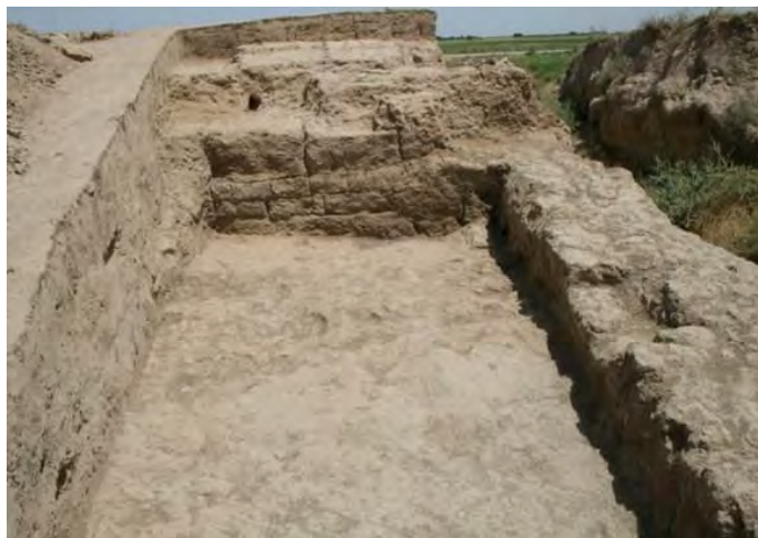
Fig. 28 - Trench no 1, SU11, Room I, with floor of a secondary occupation, after MAI, UNO, by Bruno Genito 2009
