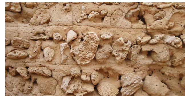
Figure 4: Wall built from coral and fossil beach rock in traditional layer technique Photo: Department of Antiquities and Museums Ras al-Khaimah.
