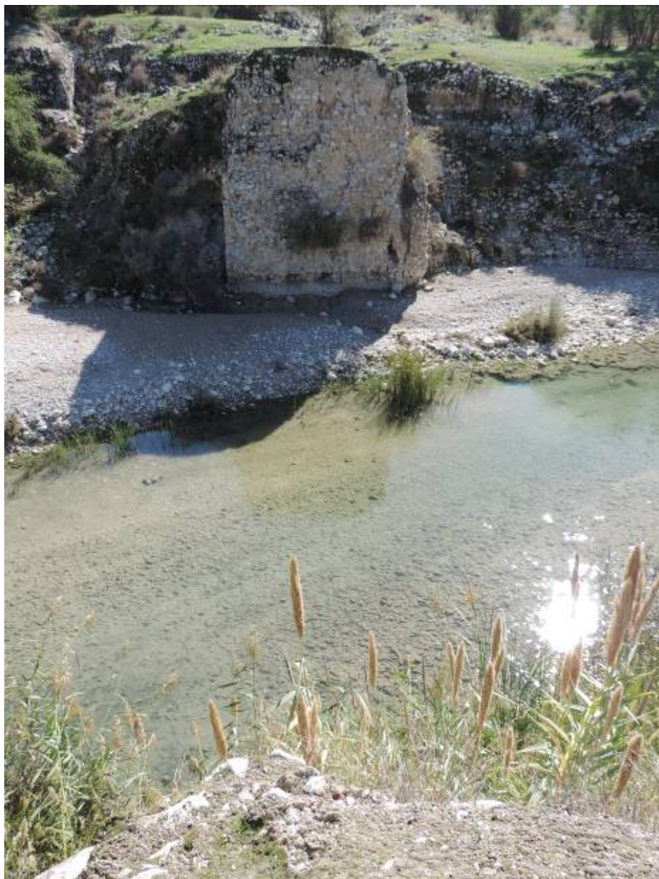
Fig. 3 - The bridge Pol-e Gabrī, as seen from right bank of the river, after MAI
