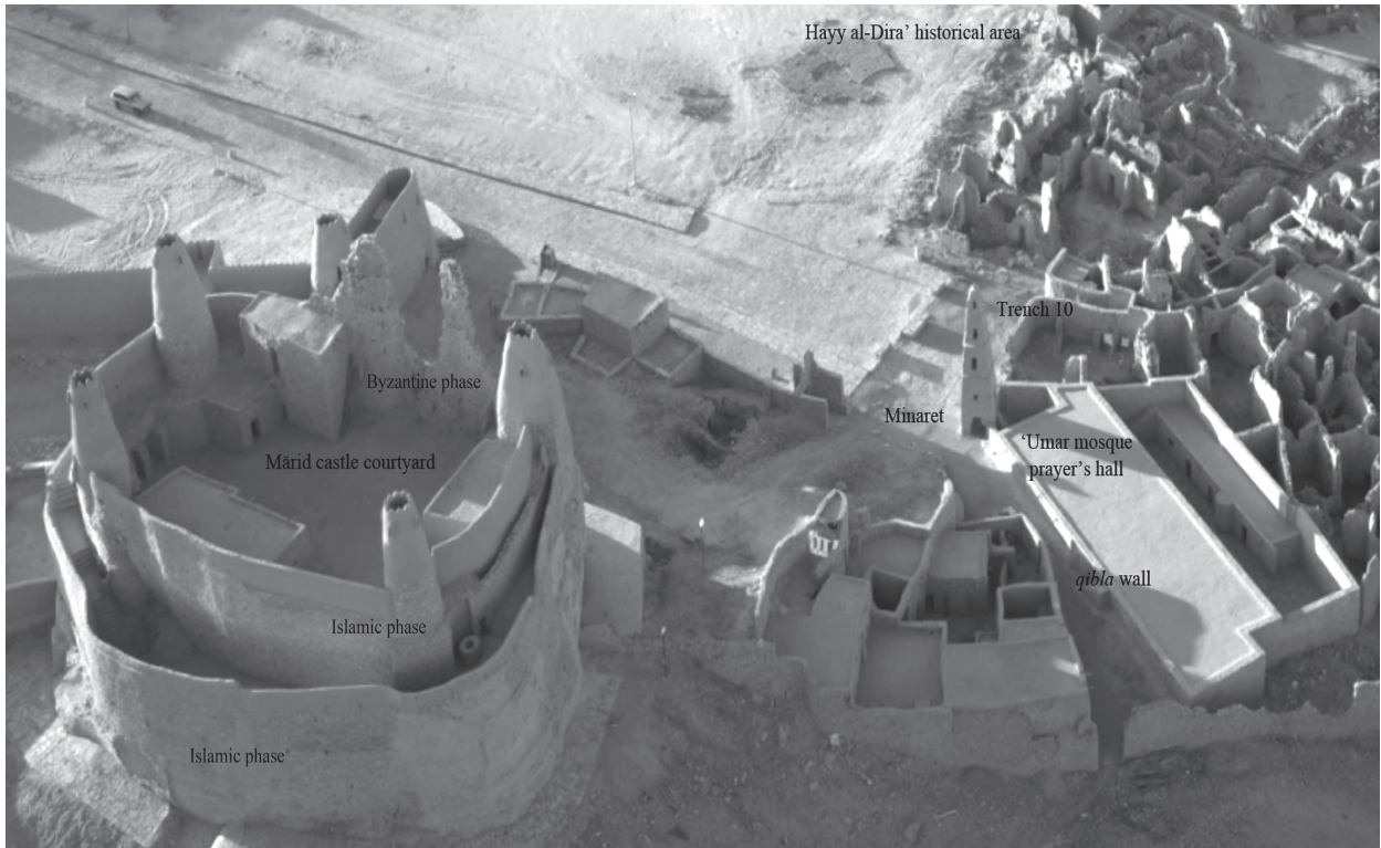
FIGURE 7. Trench 10 along the western side of the ‘Umar b. al-Khaṭṭāb mosque in the medieval historical area, view from the east (photograph Thomas Sagory, www.du-ciel.com ).
