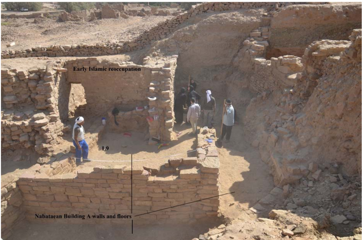
Fig. 2 - Cleaning of the Nabatean Building A floors. View from West
