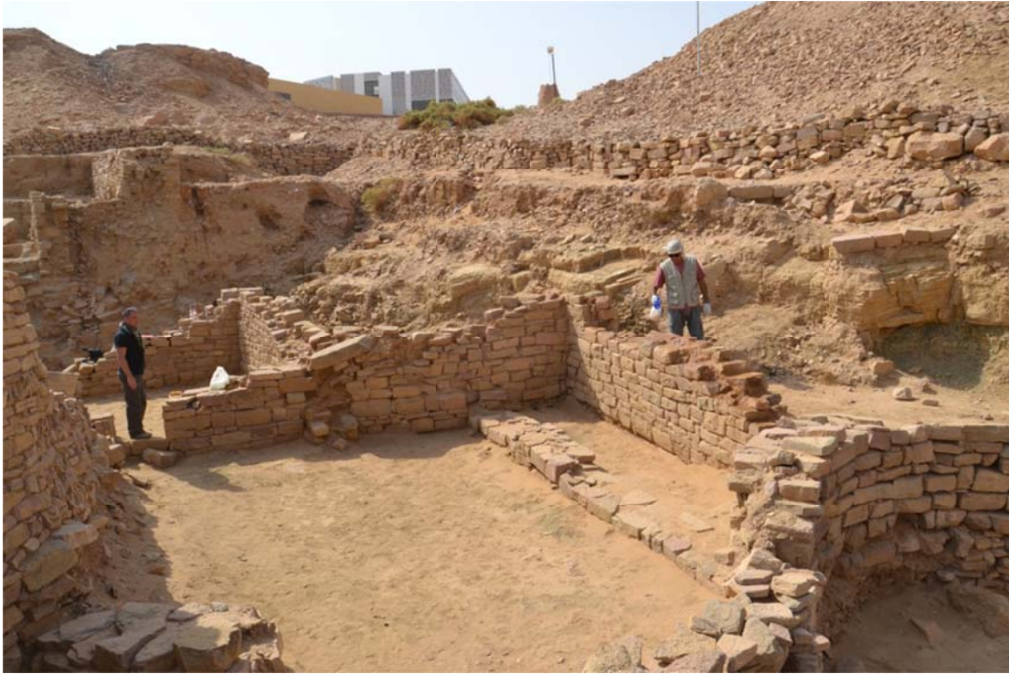
Fig. 6 - Consolidation of the upper sections of the Building A walls. View from North-East
