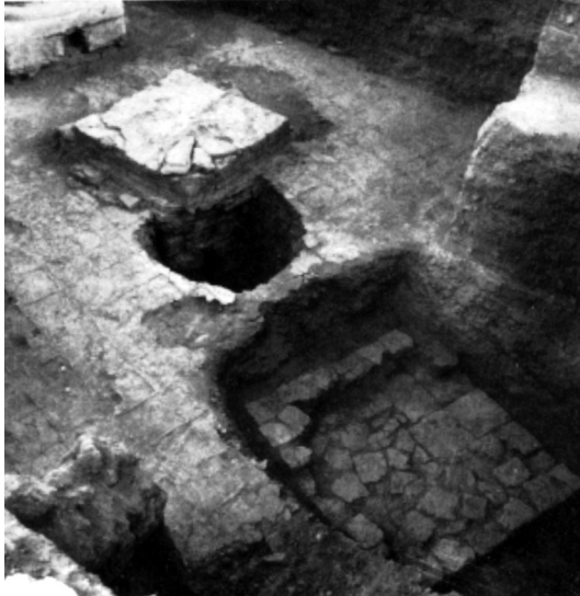
Fig. 7 – Domed hall 190, foundation of a possible second Sasanian pillar, and of the possible pillar I 2 of the 840-841 mosque; the tiled floor of a coeval building can be also seen. IsIAO Archive.
