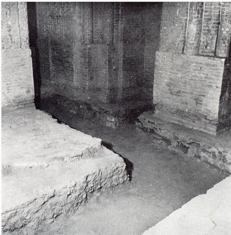
Fig. 12 – Limestone foundation of the dome of Taj al Mulk. IsIAO Archive.
