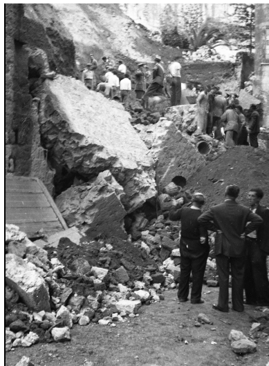
Landslide in Posillipo Photo: Archive of Riccardo Carbone
