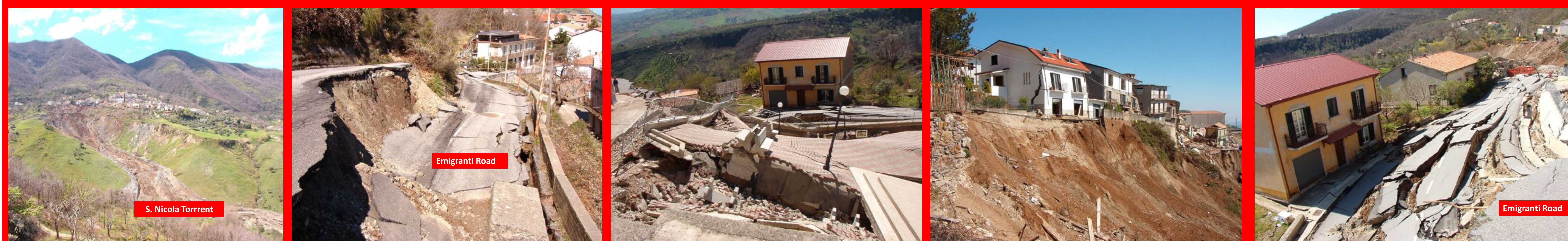
The Cavallerizzo landslide: panoramic view and damage caused to roads and buildings
