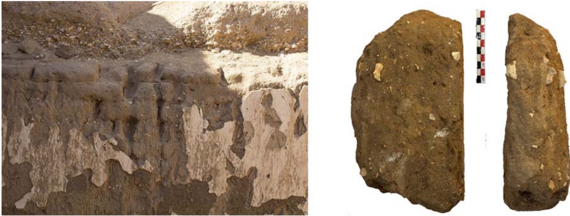
Fig. 25 - (On the left) special vault brick from AU26N, South-West wall of the underground floor. (On the right) isolated special vault-brick from the same area
