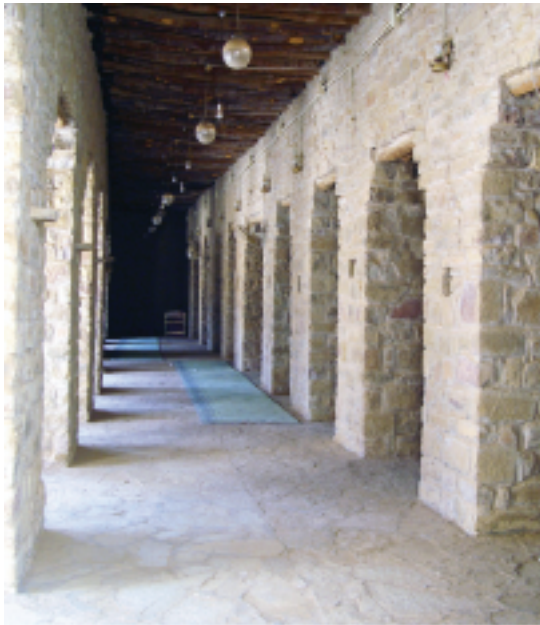
Fig. 10. The central nave of the so-called 'Umar bin al-Khattâb mosque
