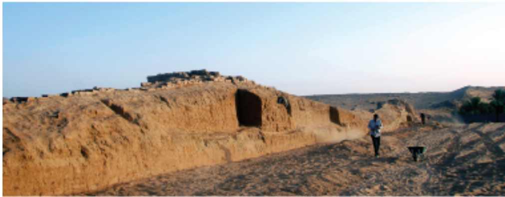
Fig. 25. The inner part of the western section of the enclosure, looking north
