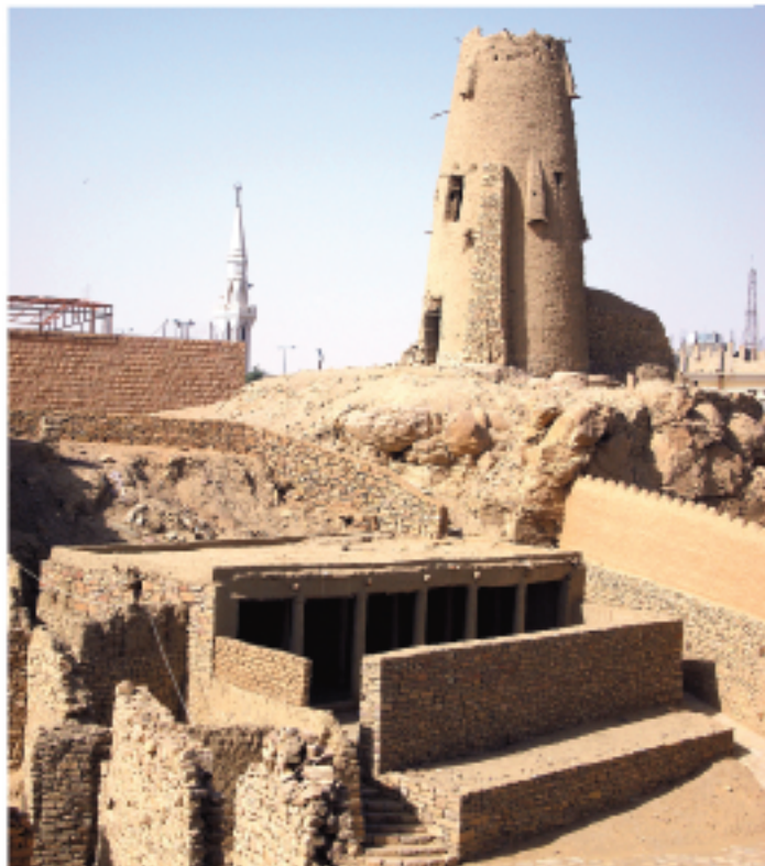
Fig. 14. Southern annexe of the Qasr Mârid, looking south
